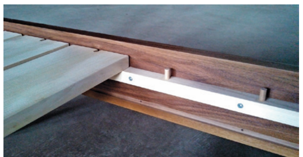
Figure 8: Ledger board and slats
